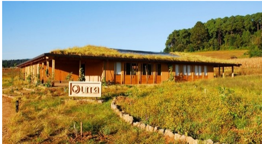
Figure 49 UMA access road https://umamexico.com/wp-content/uploads/2019/11/EntradaUMA.jpg
