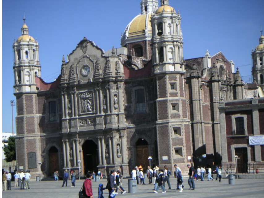
Figure 27 Restoration Efforts Aim to Save the Sinking Basilica Guadalupe in Mexico City. Photograph by Jay Peebles / Flickr
