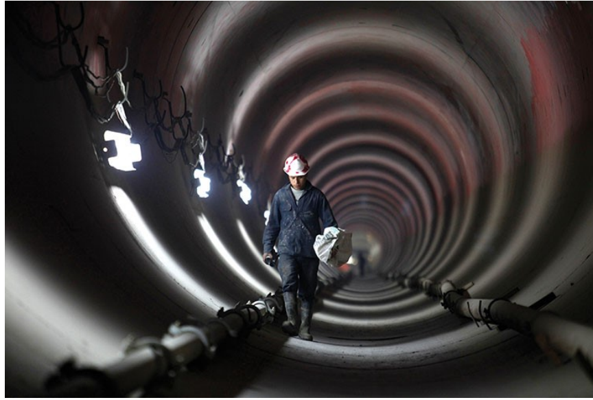
Figure 31 A worker inside one of the tunnels that make up Mexico City's deep-drainage system. (Photo by Dario Lopez-Mills/Associated Press. )
