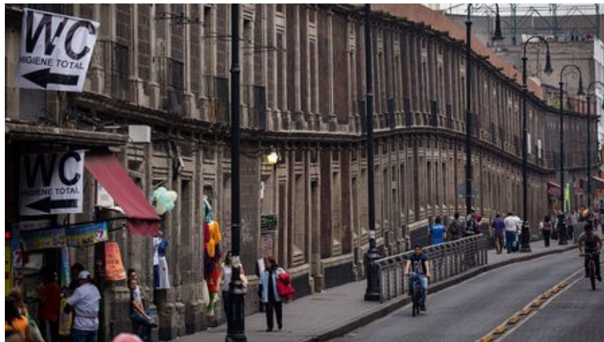
Figure 25 As Mexico City sinks, its structures twist and deform. JOSH HANER/THE NEW YORK TIMES
